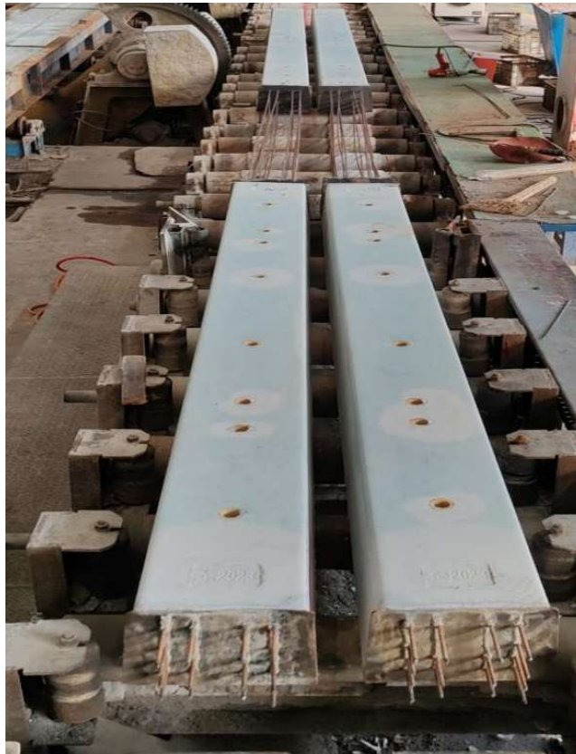
Fig. 19. Steel bars for rail sleepers to be cut
